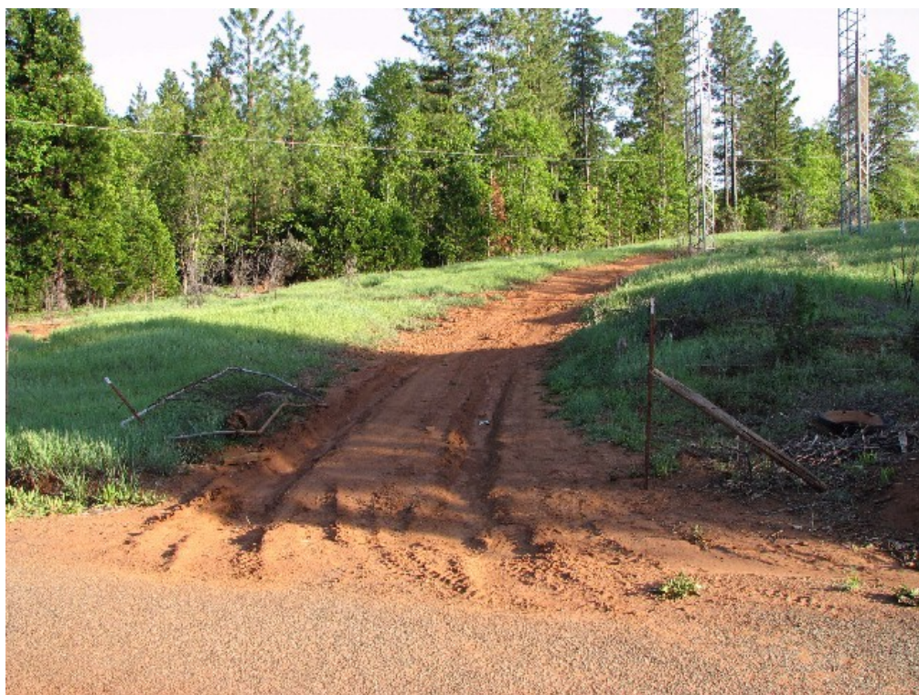
Transmission Corridor access road, erosion flowing onto county road, May 2009, Oak Run.
