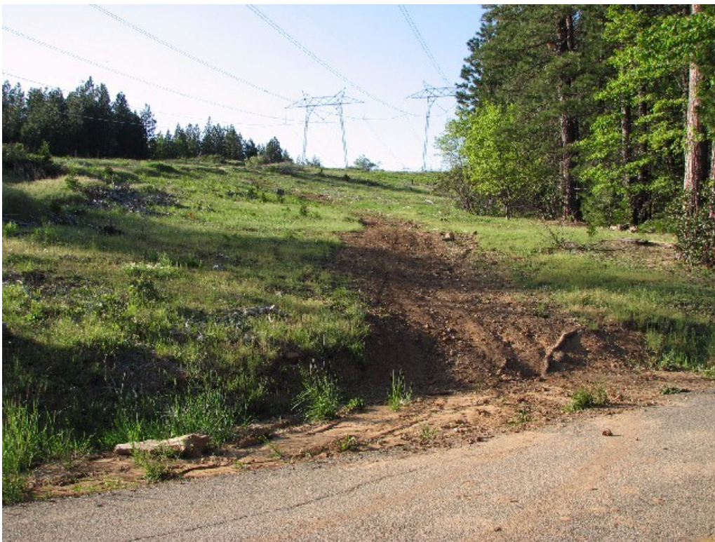
Transmission Corridor access road, erosion filling drainage ditch and flowing onto county road, May 2009, Oak Run.
